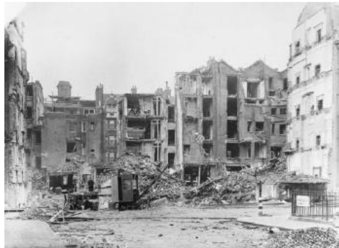
Damage to St Bartholomews Hospital
